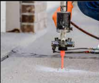
CONCRETE LEVELING
